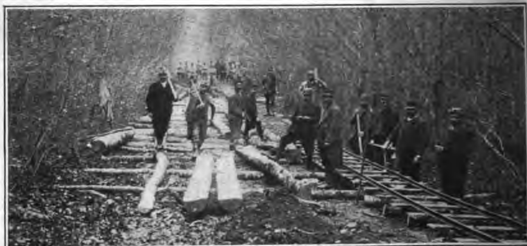
LOGS QUICKLY BECOME CROSS TIES, AND THE RAILS ARE LAID
